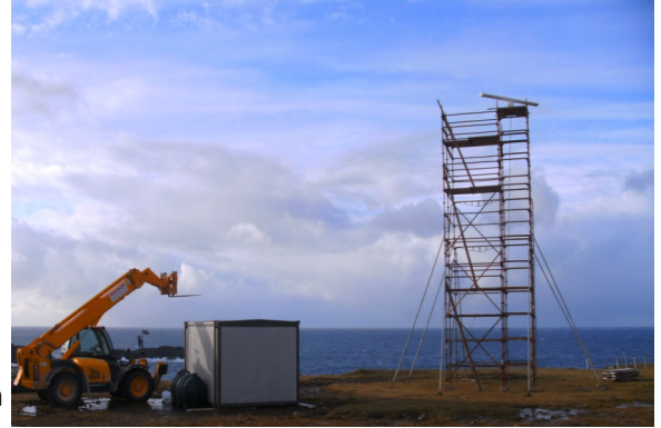
Construction of survey station on cliff tops near Belmullet
